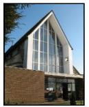
The west end of the Church had never been properly completed. This created a problem as it was exposed to the prevailing winds and rain. The original structure of lath and plaster with tiles to the exterior was not adequate and was blown in during gales in the 1960s. (How dark the Church must have been when it was lit only by gas until electricity came in in the 1920s).
